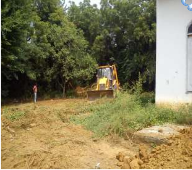
Construction /Landscaping of School in Progress
