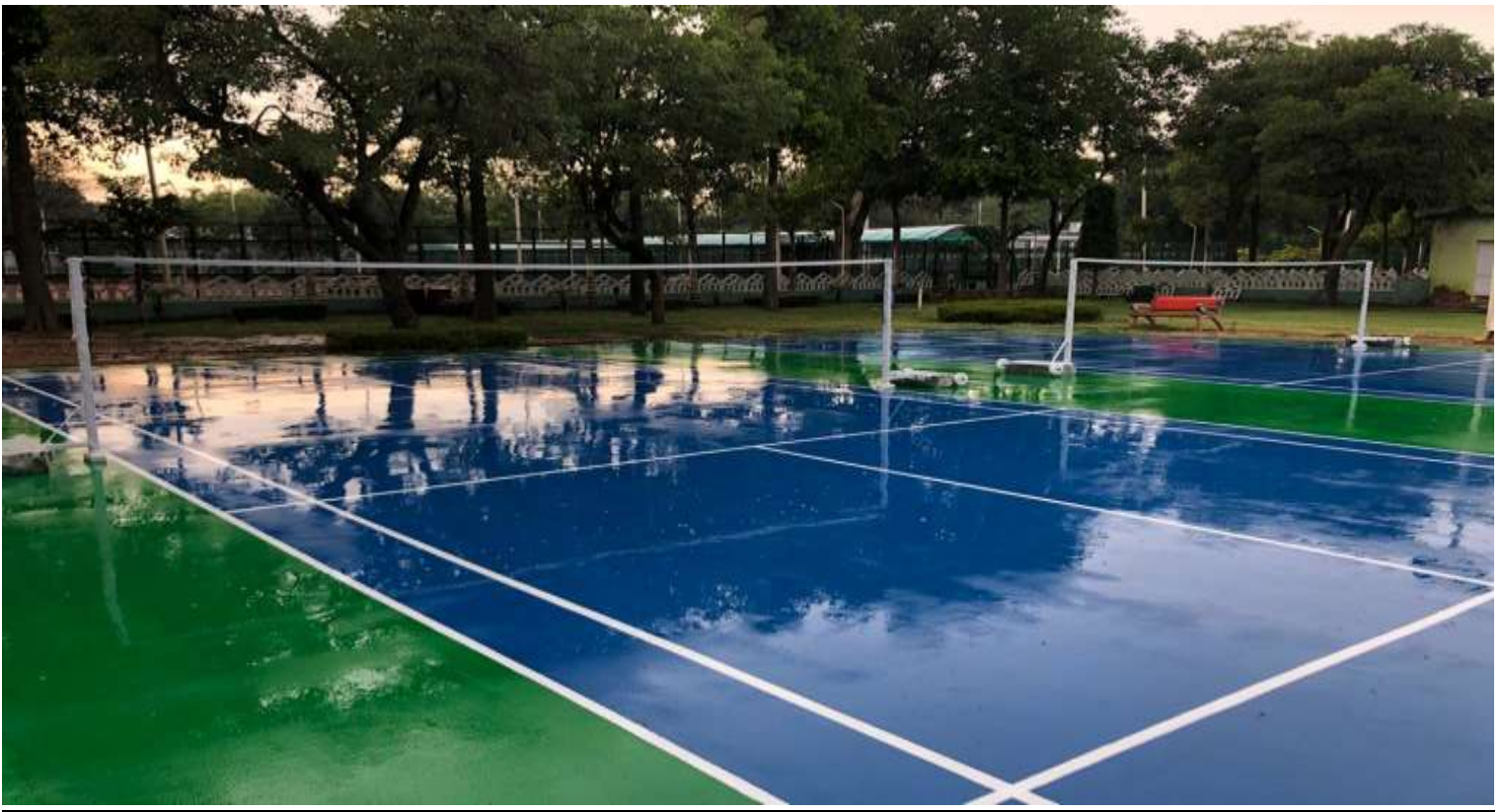
Badminton courts on completion in Paschim Vihar Sports complex DDA
