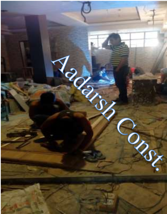
Residential Construction work in Progress
