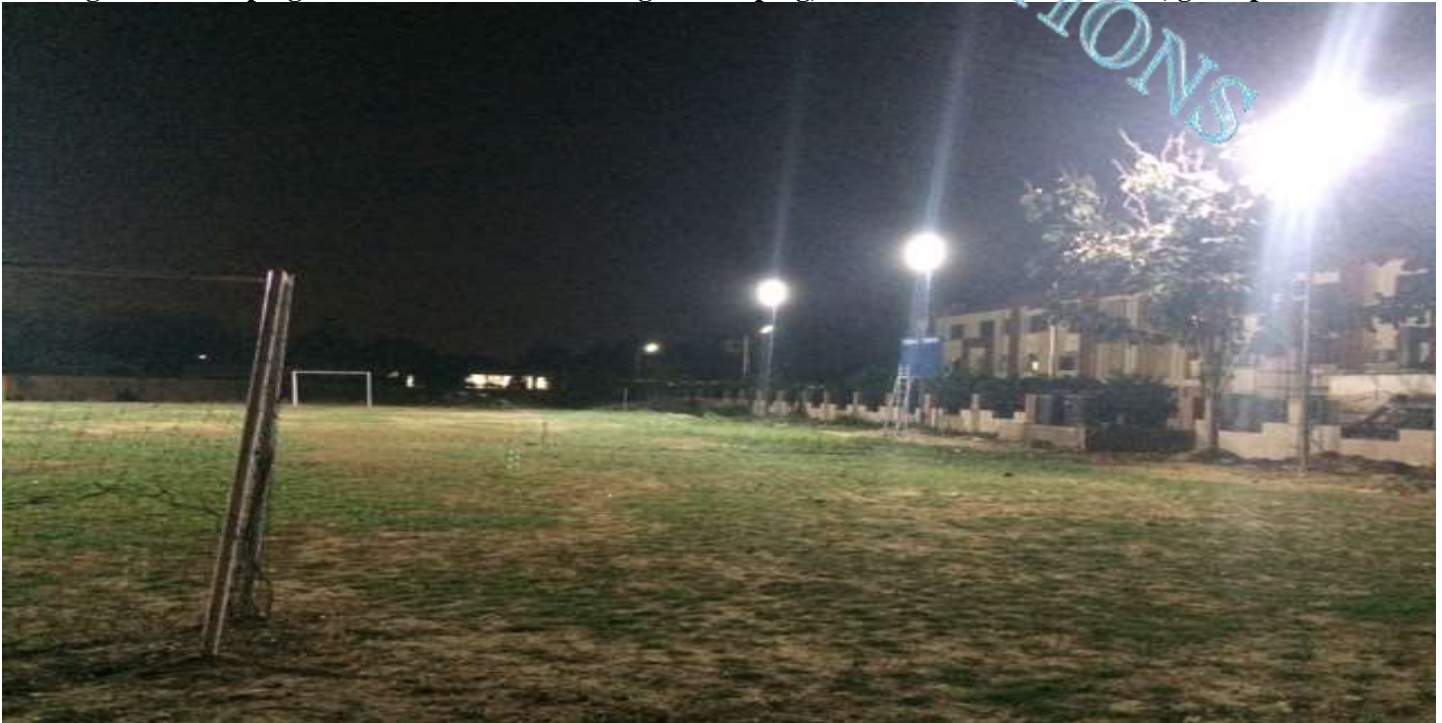
Picture of Same Field On almost completion stage , flood lights installed, horticulture completed and grass catching roots at Air Force Head Quarters, Palam
