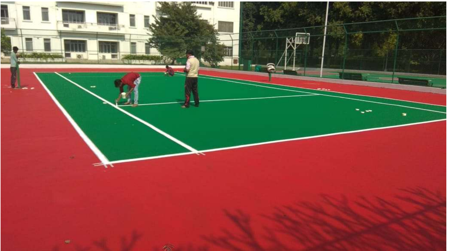
LAWN TENNIS COURT ON COMPLETION IN A SOCIETY IN NOIDA
