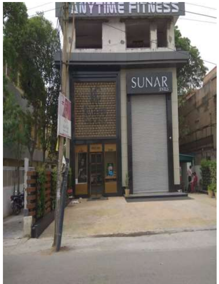
Picture of place at completion of entire work
