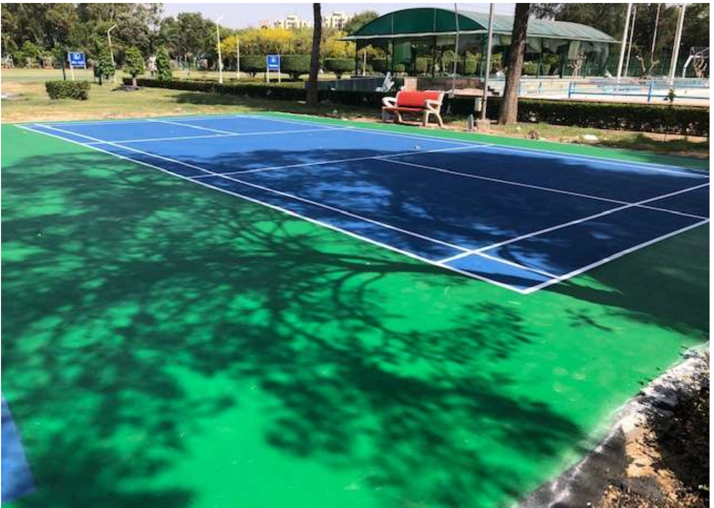
Work completed DDA sports complex synthetic courts, Rohini
