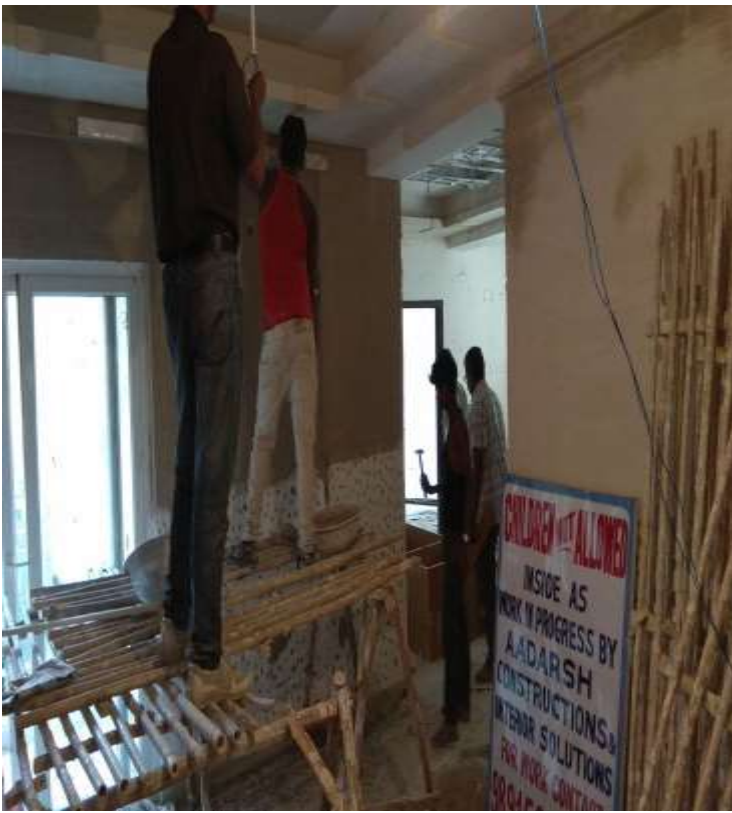
Work of Drawing Room in Progress
