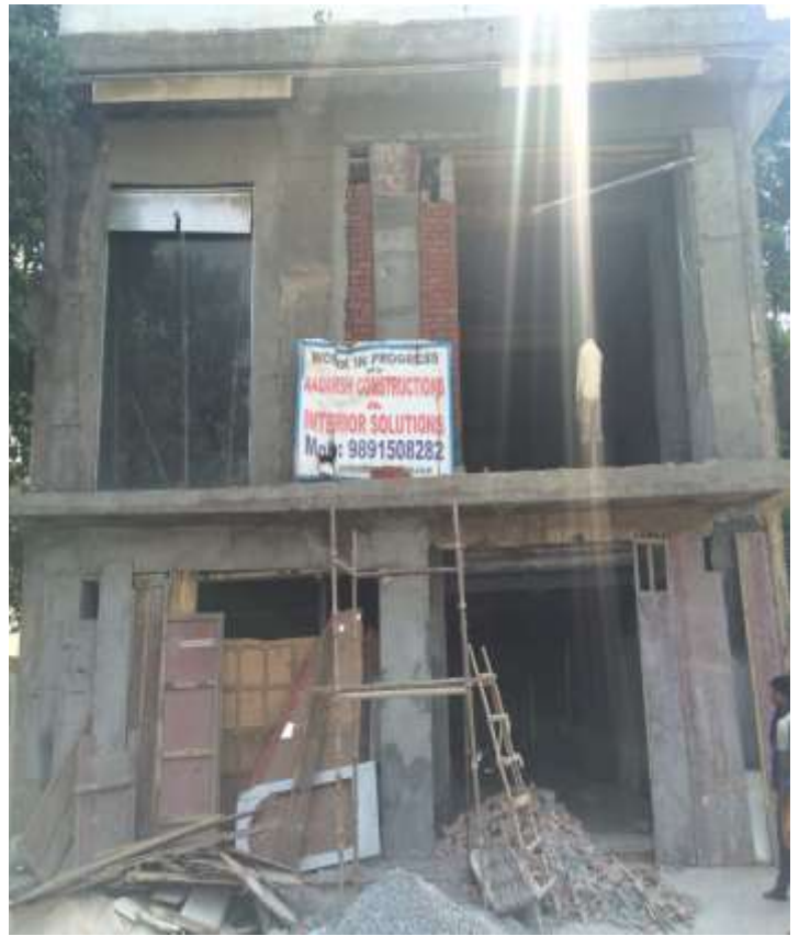
Picture of work in Progress
