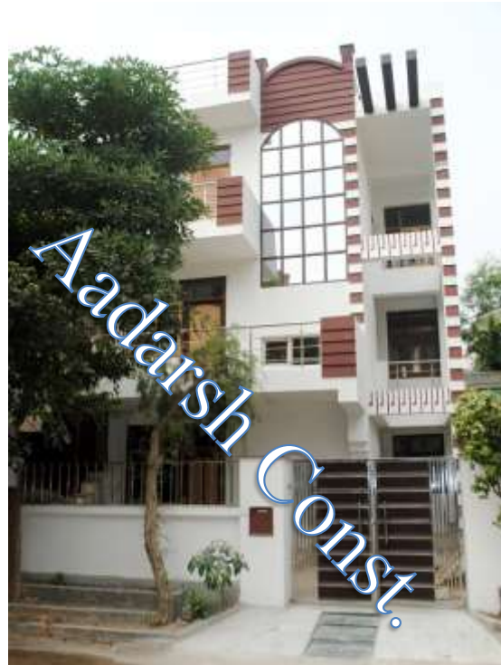
After Completion of residential Project, Gurgaon
