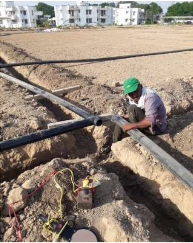
Sprinkler work in progress ,installation and commisioning at cricket ground
