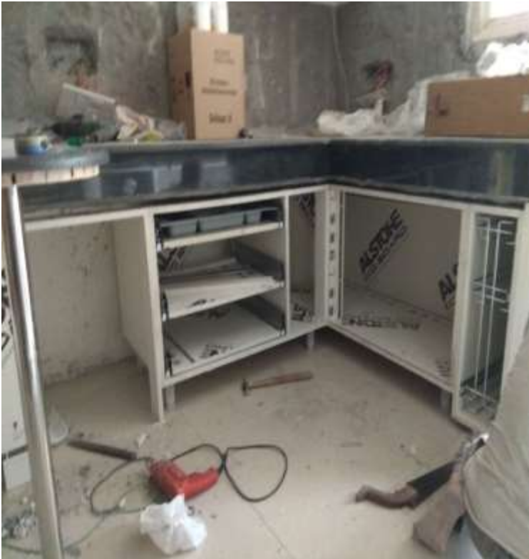
Work of Dining and Kitchen in Progress
