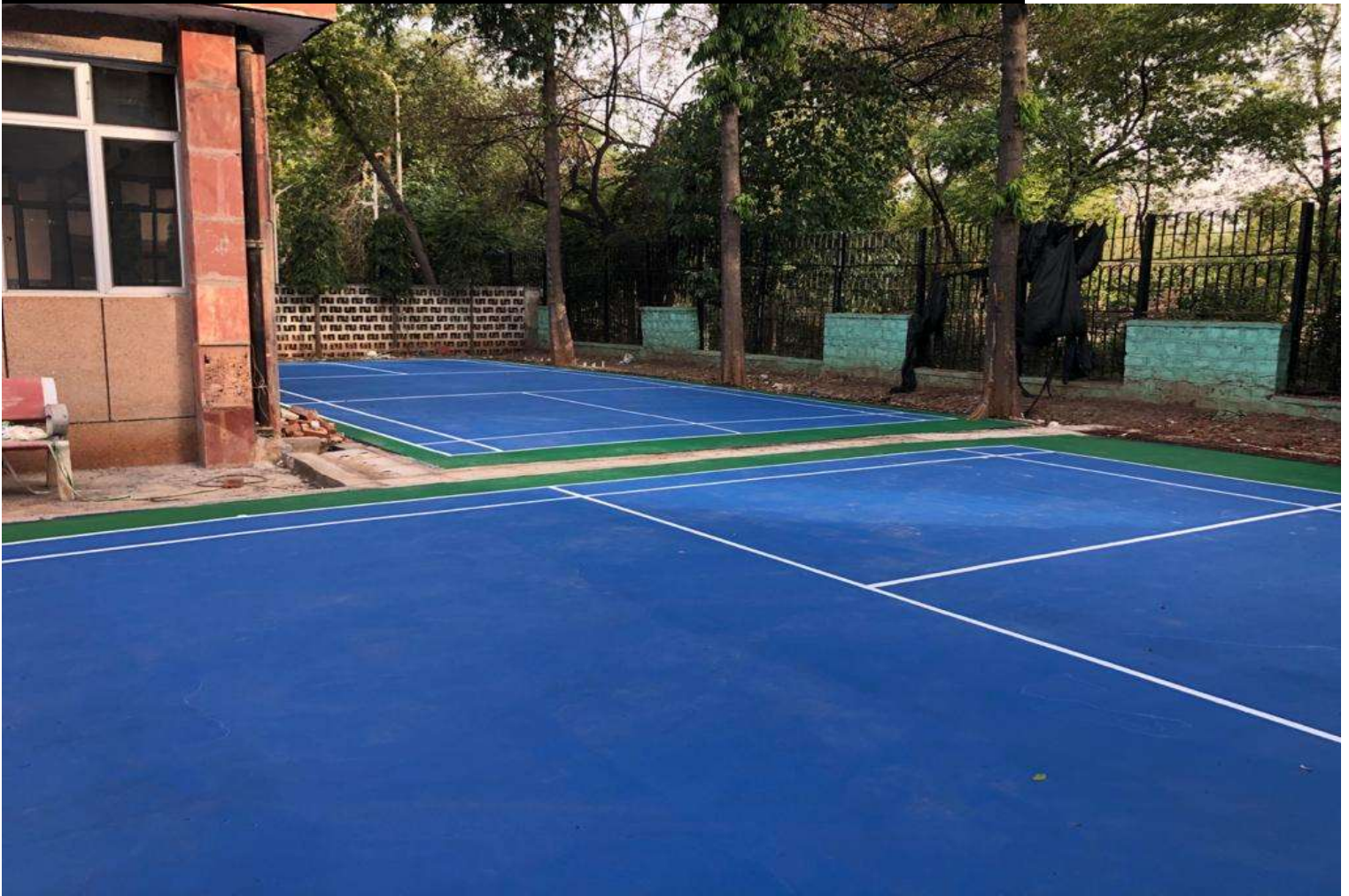
BADMINTON COURTS ON COMPLETION IN SOCIETY IN GURGAON
