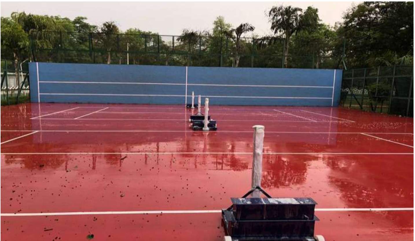
DDA SPORTS COMPLEX ROHINI LAWN TENNIS PRACTICE COURTS ON COMPLETION
